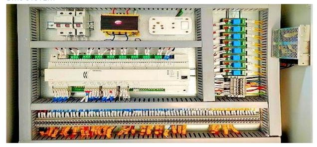
A building management system (BMS) is a control system that can be used to monitor & manage the mechanical, electrical and MEP services in a facility. Such services can include power, heating, ventilation, air-conditioning, physical access control, pumping stations, elevators and lights.
